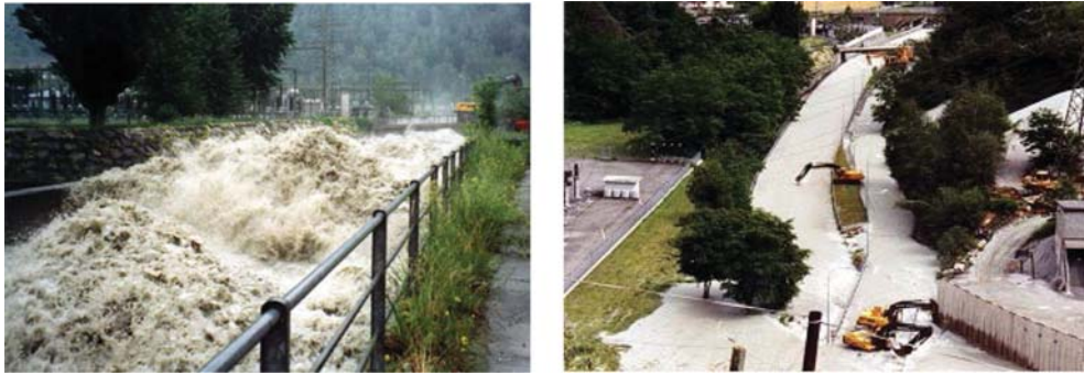
Figure 6. Left: Surface waves due to anti-dunes regime during sedimentation in the flushing channel. Right: High sediment load leading to channel overtopping in 1999.
