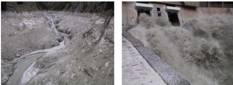
Figure 4. Flushing operation 2003. Left: Erosion and transport process in the reservoir after complete drawdown. Right: Fluid-solid mixture downstream from the bottom outlet during a flushing operation.
